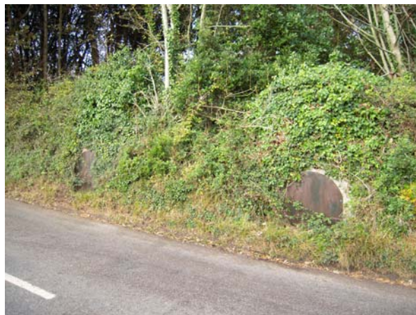
Figure 6: The lime kilns, under heavy overgrowth.
