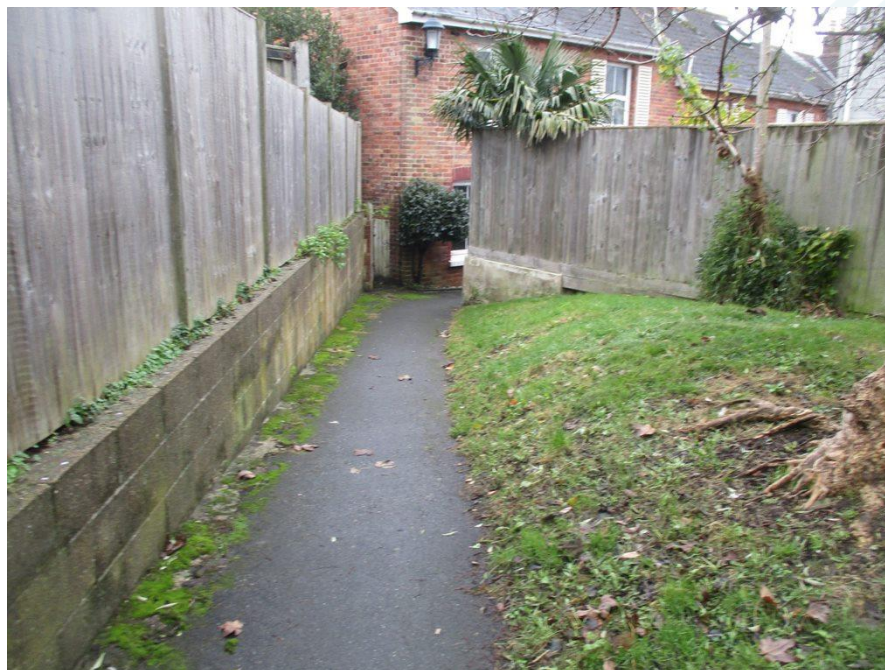
Figure 8-6: Location 2, footpath between Kings Road and Station Road.
