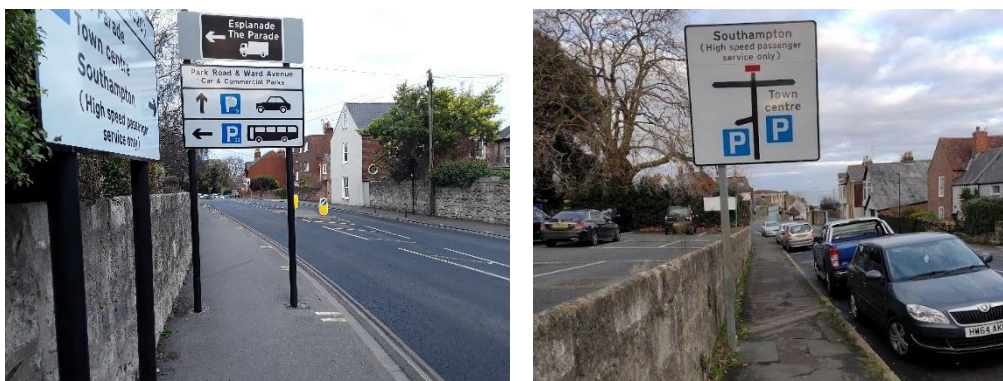
Double pole sign (left) obstructs the footway. Cantilever sign (right) leaves footway clear
