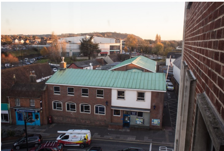
Figure 7: Newport Police station.
