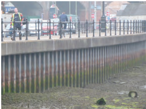
Steel Sheet Piling
