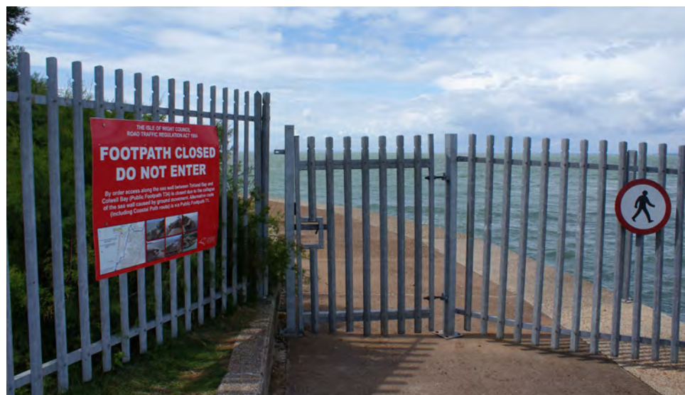
Coastal access severed due to the landslide at Totland in 2012
