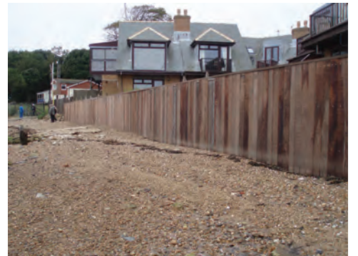
Timber Clad Sheet Pile Wall
