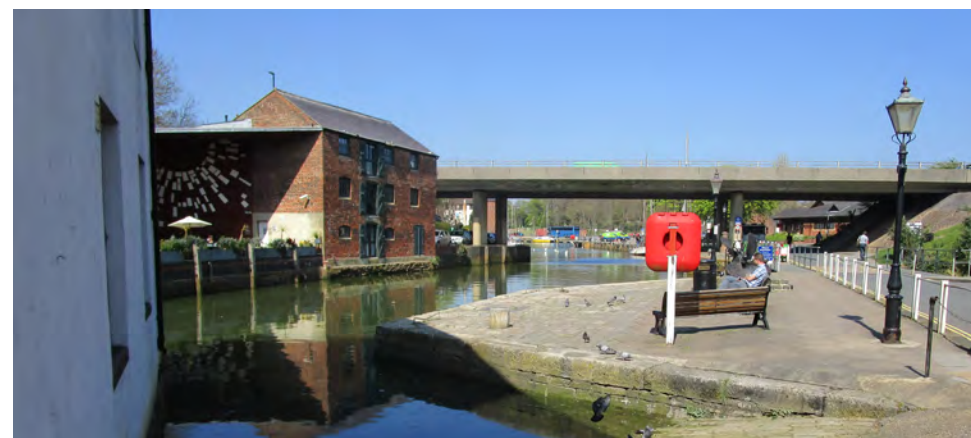
Quay walls of Newport Harbour
